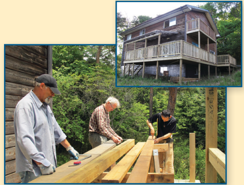
Volunteers working hard rebuilding our decks.
