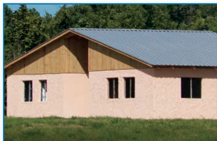
Men's dorm completed with new roof.
